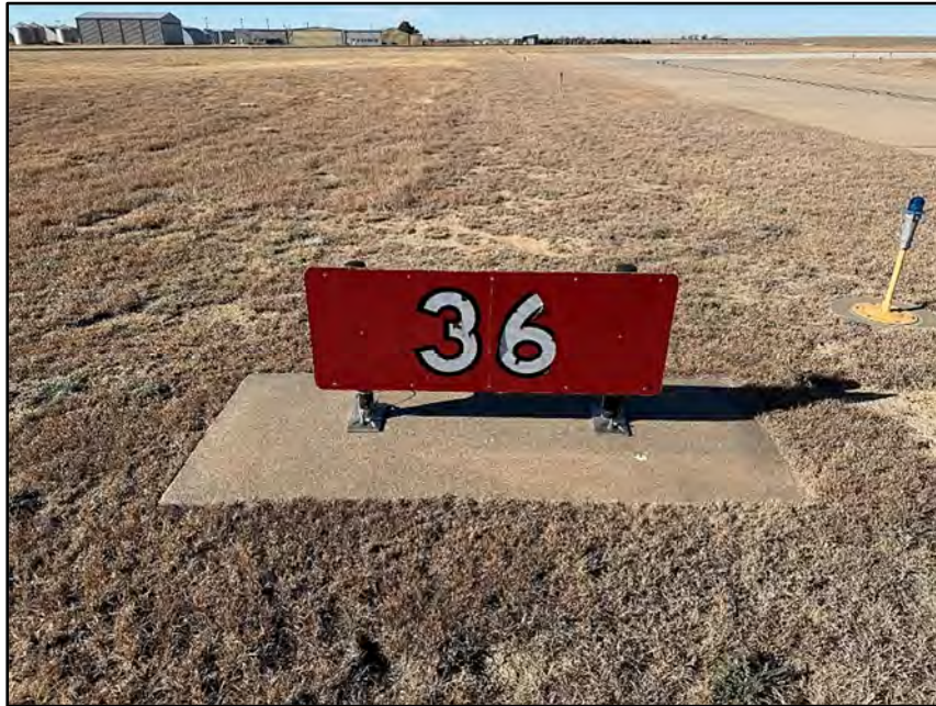
Figure 3: Existing Non-lighted Runway Holding Position Sign
