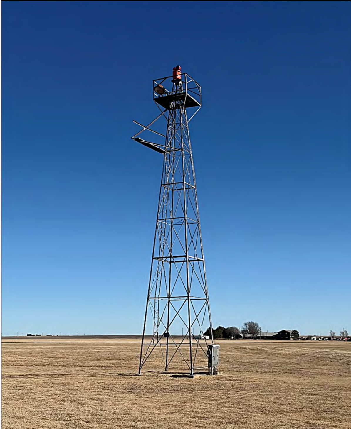
Figure 8: Existing Beacon and Tower
